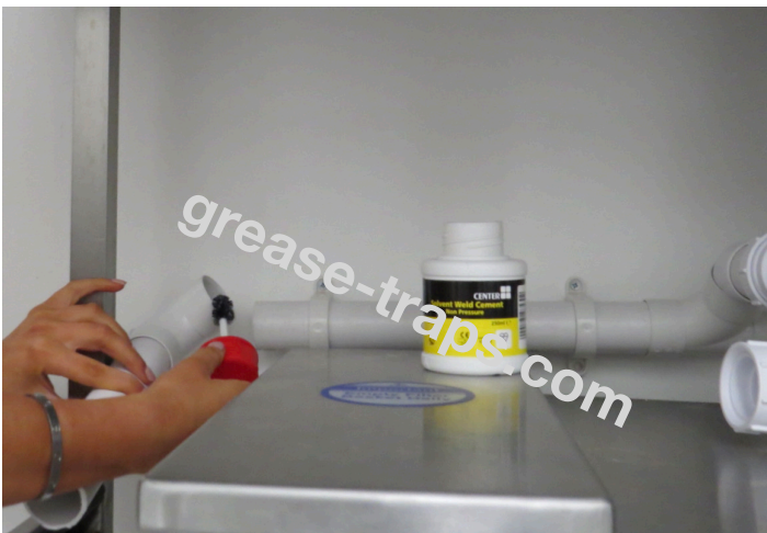
Glue Pipe Work Using Solvent Weld Adhesive
