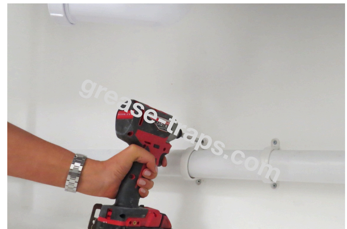
Secure Pipework To Wall Using Brackets
